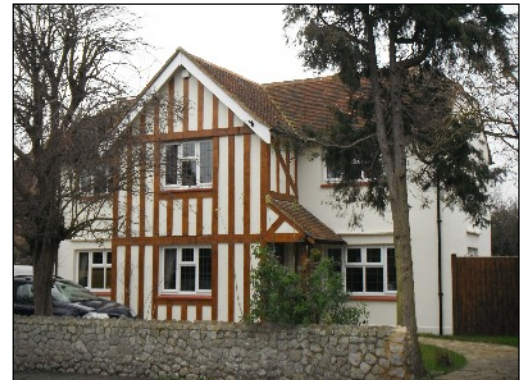
4 Bridge Road, Westbrook (Renovation)
