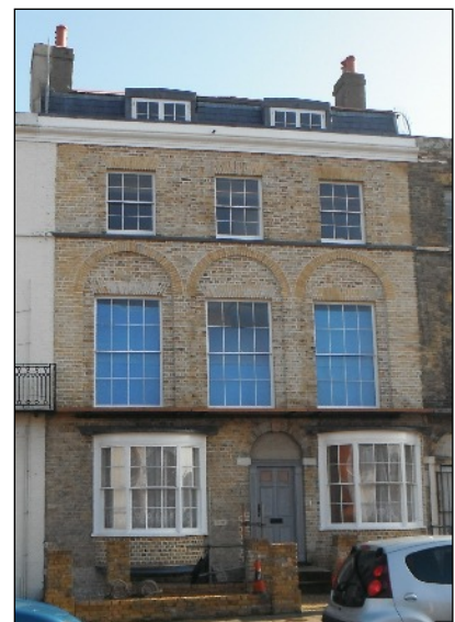
12 Zion Place, Cliftonville (Renovation)
