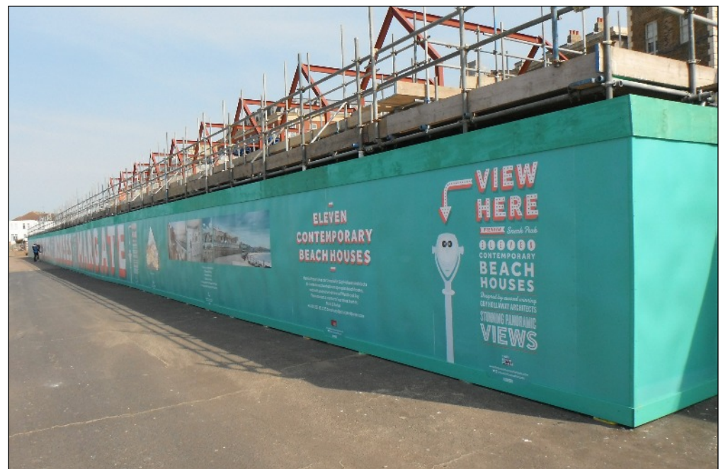
Another view of the temporary hoarding alongside the promenade at Westbrook Bay with members of the public taking the opportunity to view the works
