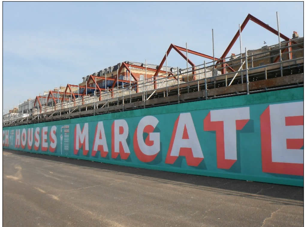
The temporary hoarding alongside the promenade at Westbrook Bay
