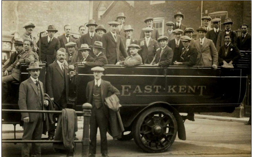
Note the railings on the left of the picture
